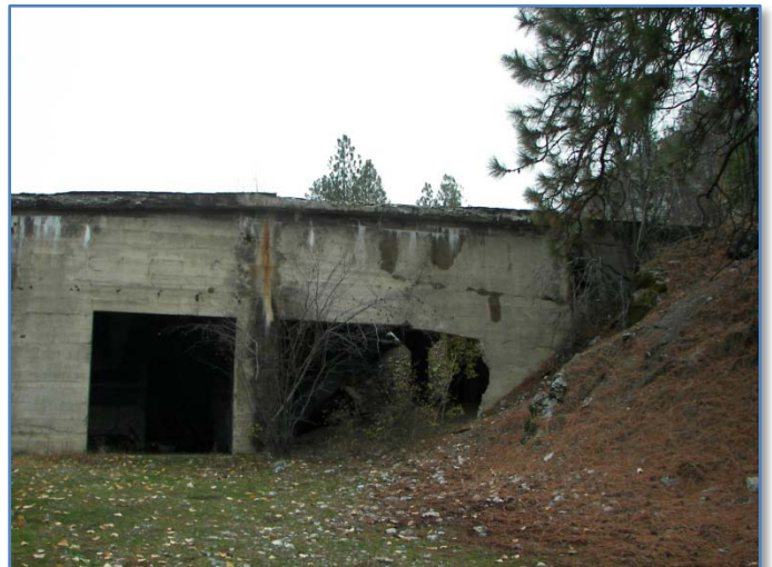
The Rock Crusher and Townhouse Suites building. Photo by Vince Rundhaug.
